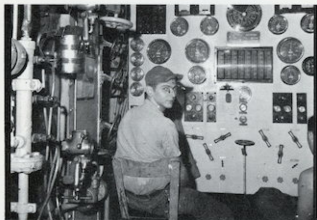
No sir, this isn't #1 pump room
